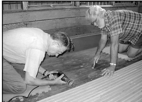
Don Hulse (left) and Rich Berens prepare the floor of the No. 25 prior to painting and seat installation. – Photo © Darrell Arndt.
